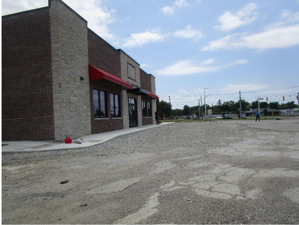
View of site looking south
