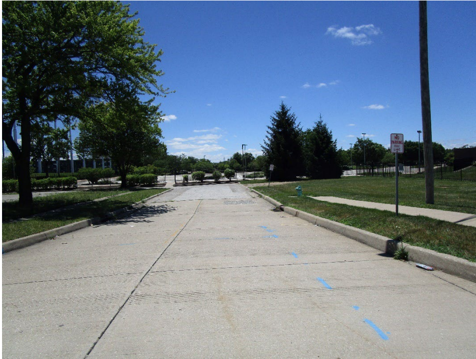
View looking south along Bridge Street
