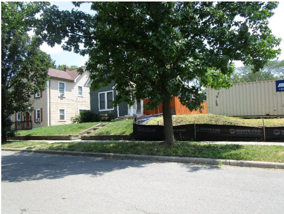
View looking of site and adjacent single-family dwelling northeast across North Jefferson Avenue
