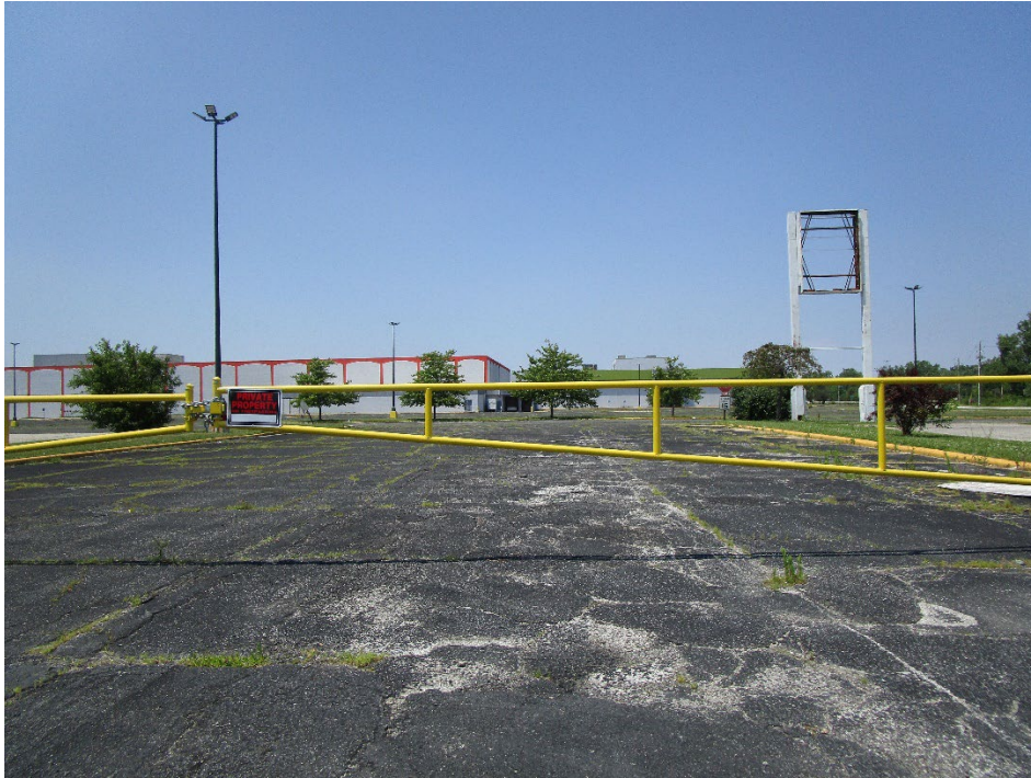
View of southern portion of site looking north
