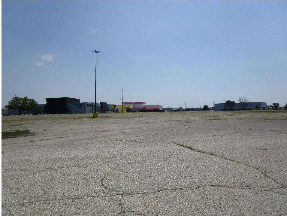
View of central portion of site looking south
