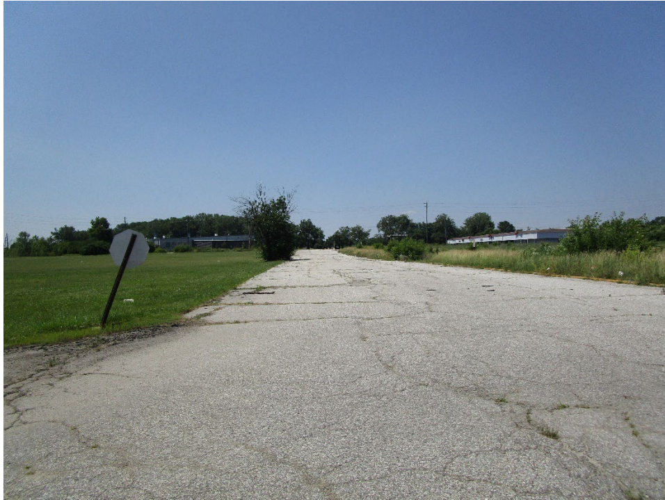
View looking north along Century Plaza Road internal to the site
