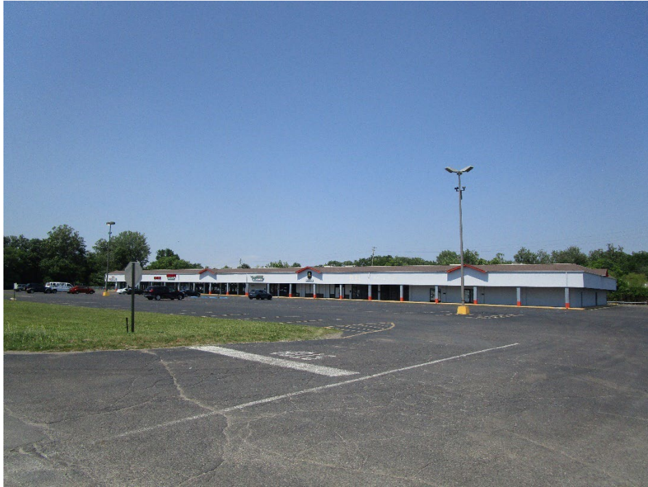
View from northern portion of site looking northeast
