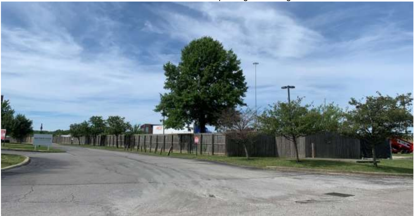
Photo of the existing fence between the subject site and apartments to the east.
