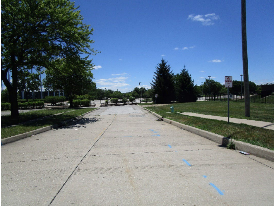
View looking south along Bridge Street
