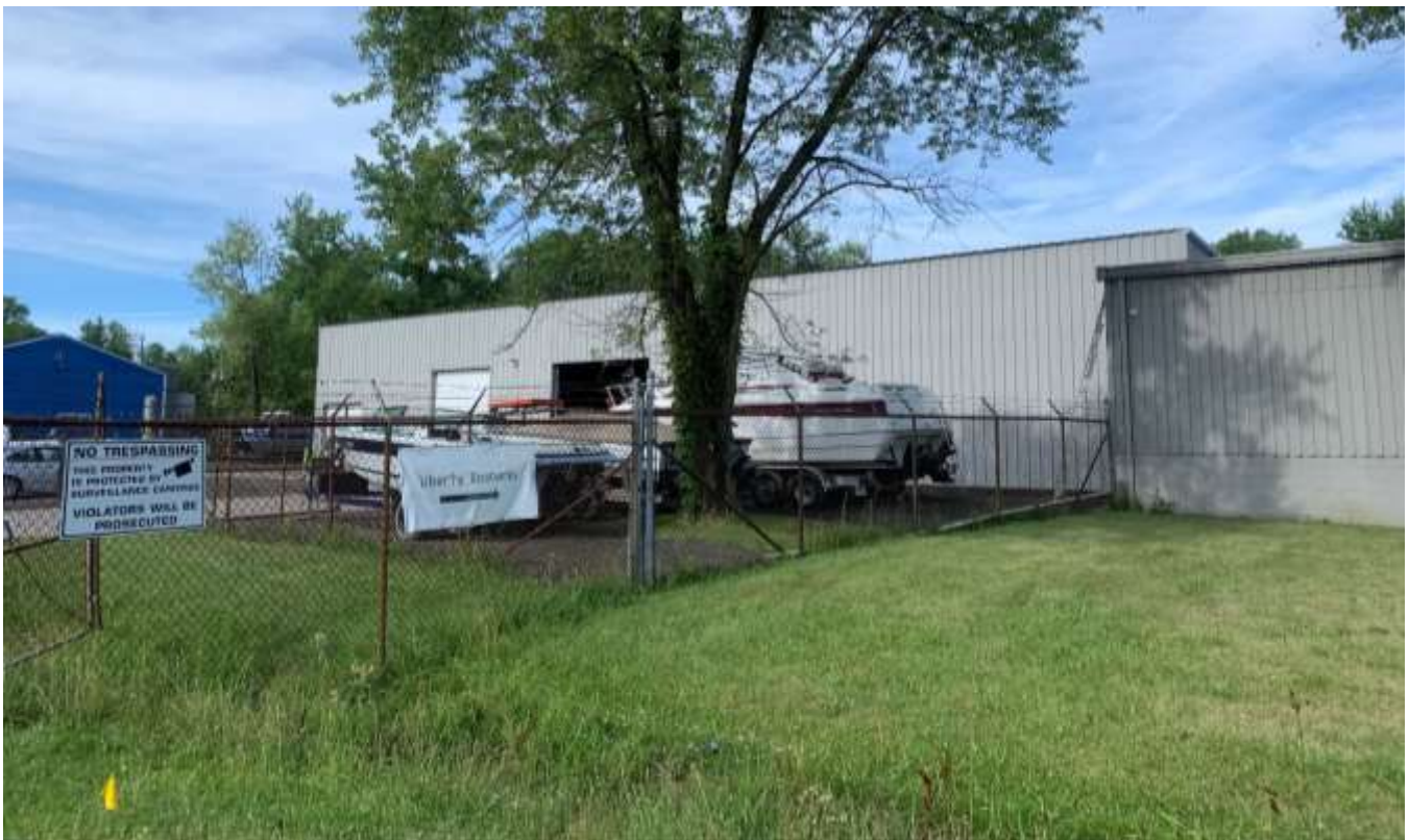
Photo of the fenced in area east of the building.
