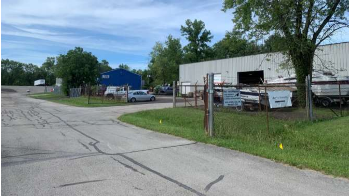
Photo of the fenced in area east of the building that leads to the rear of the site.
