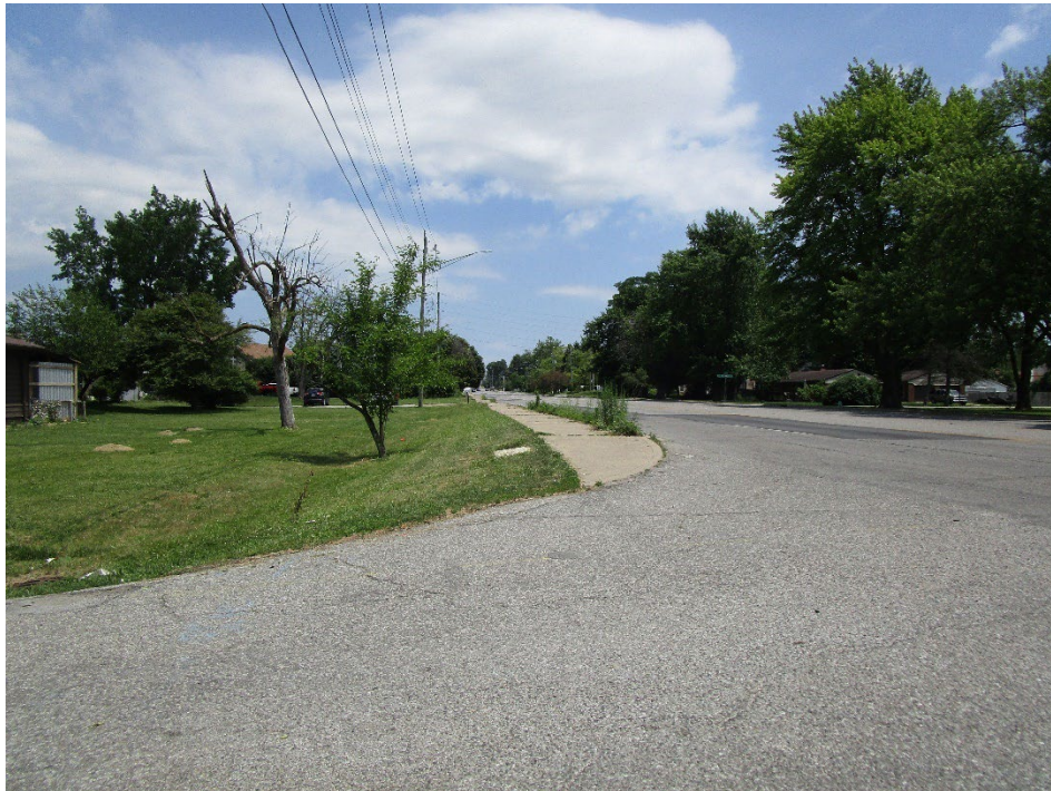
View looking east along East Stop 11 Road
