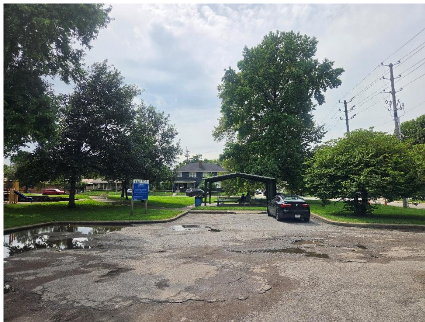
Photo 2: Existing Shelter Viewed from East
