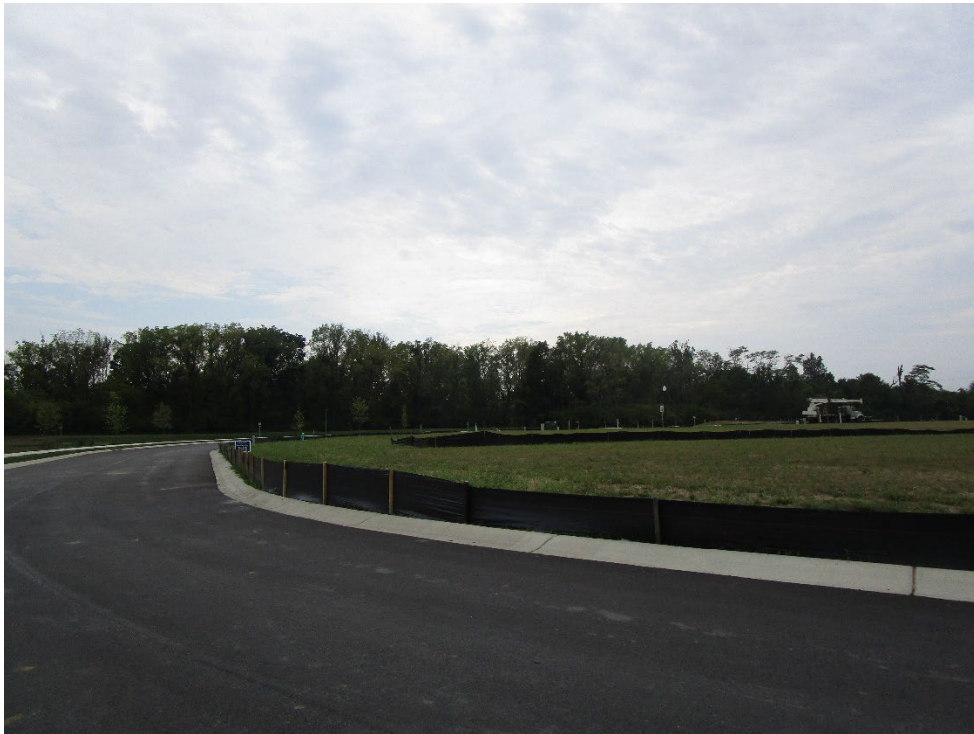
View of site looking southeast across Everland Place
