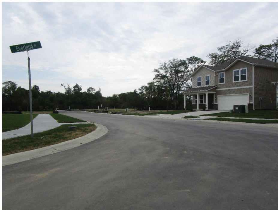
View of site looking southeast
