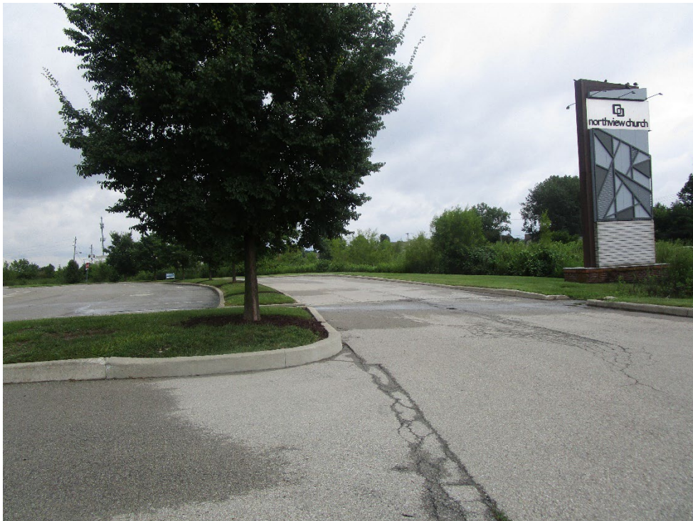
View looking east along Northview Way
