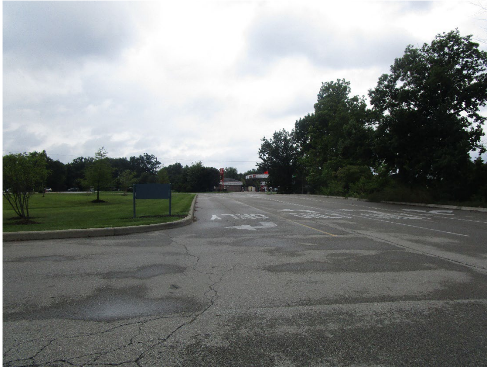
View looking south along Northview Way
