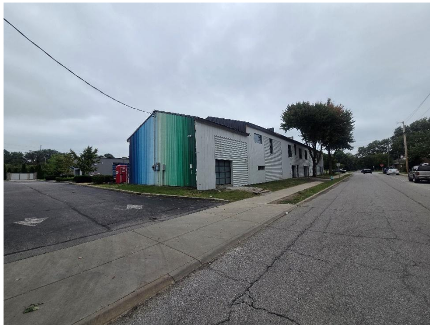
Photo 4: Western Building Viewed from Northwest
