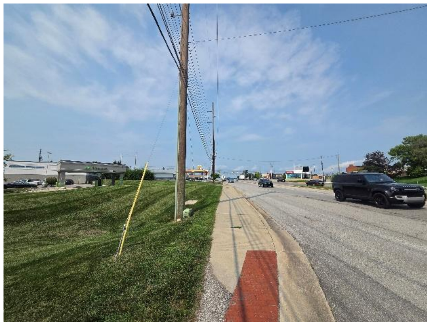
Photo 10: Allisonville Road Existing Sidewalk from South
