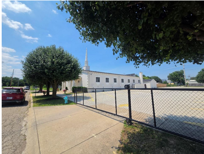
Photo 9: Existing Building on 1540 Ohio and 211 Reisner
