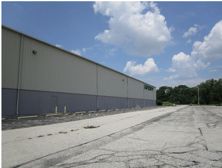
View of site looking north
