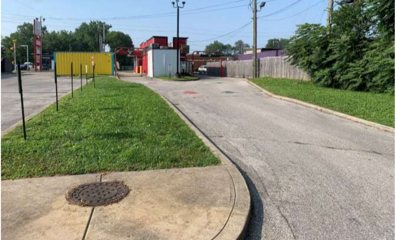
Photo of two one-way lanes for pick-up and ordering looking south.
