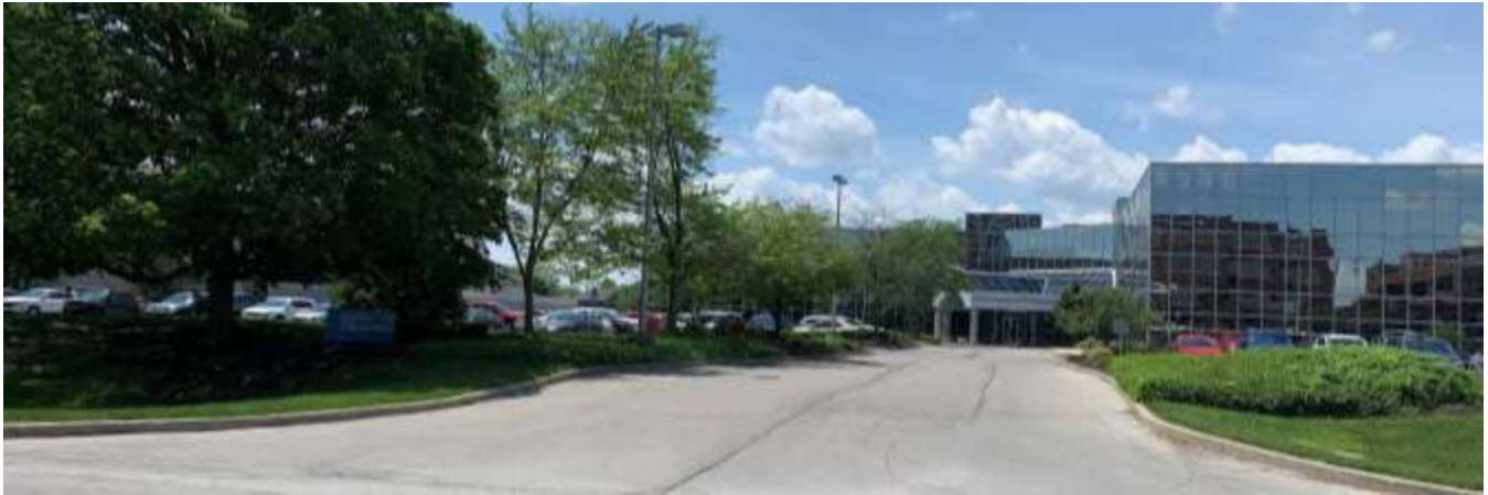
WF20 to be replaced along Naab Road.
