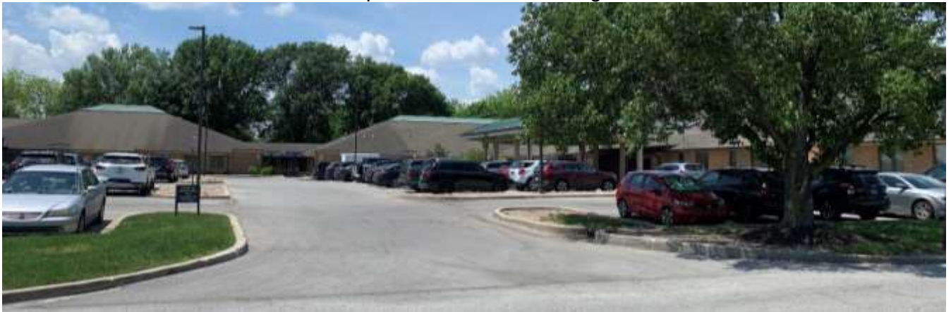
E18 to be replaced along Naab Road.
