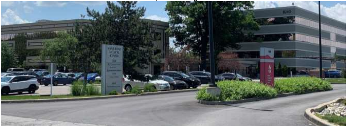
WF21 to be replaced along Naab Road.
