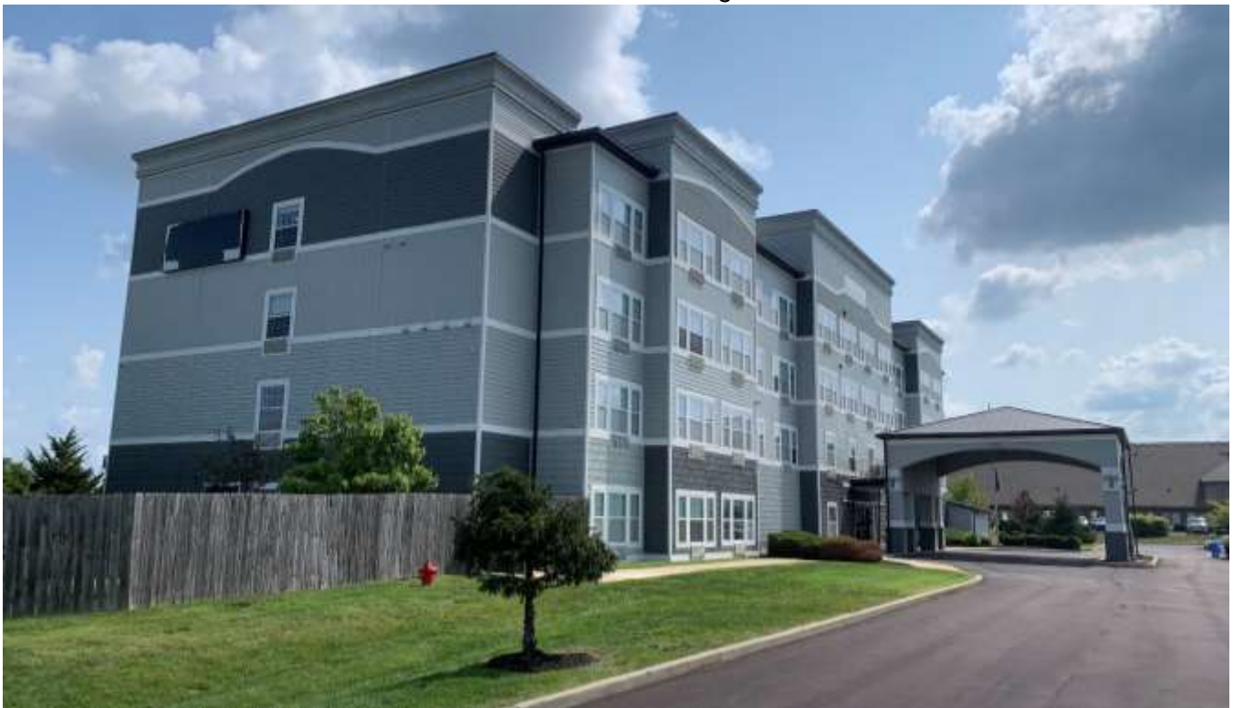
Photo of the eastern building façade.
