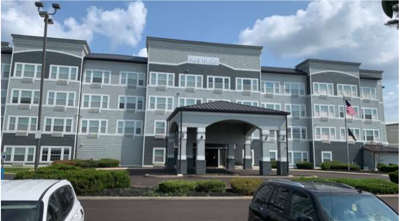
Photo of the southern building elevation.
