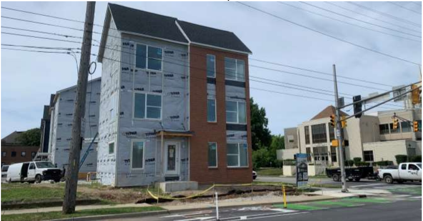
Photo of townhomes west of the site.
