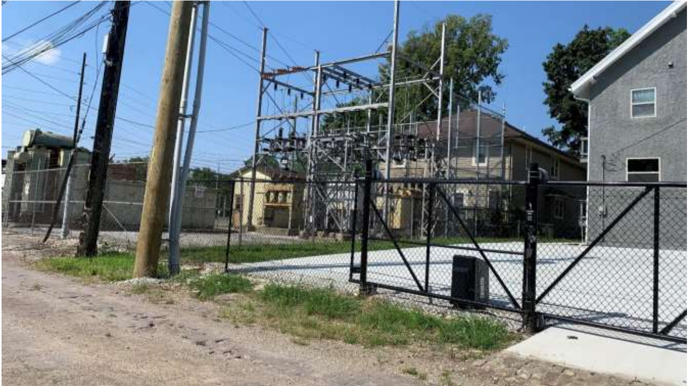
Photo of the grass area south of the parking area and adjacent electrical substation.
