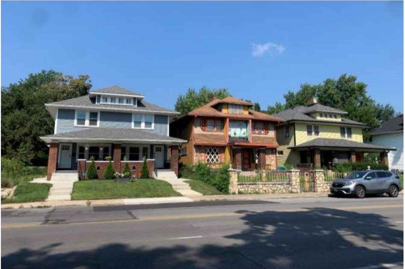
Photo of two-family dwellings west of the site.
