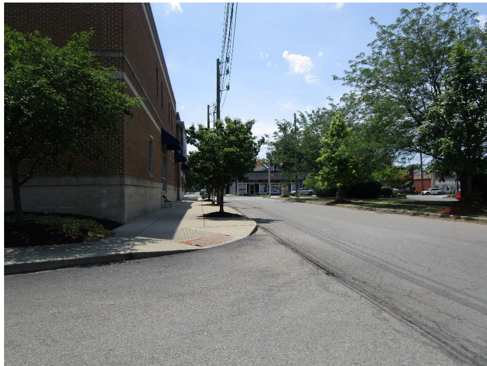
View looking south along North Jefferson Avenue
