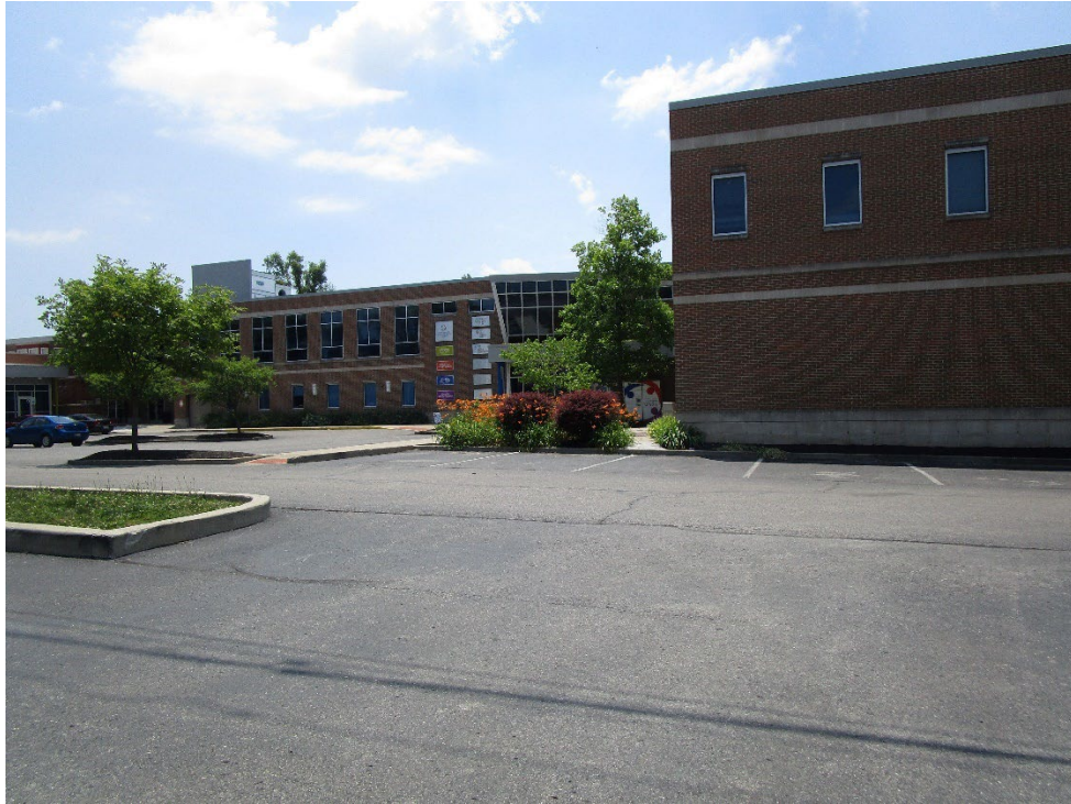
View from site looking southeast
