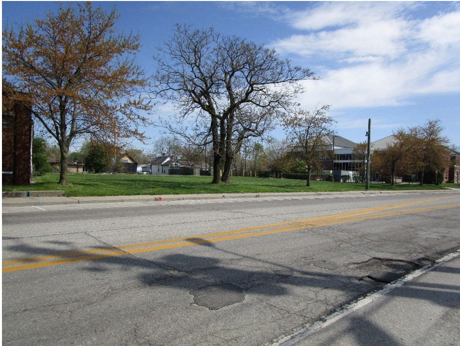
View of site looking southeast across Dr. Martin Luther King Jr. Street
