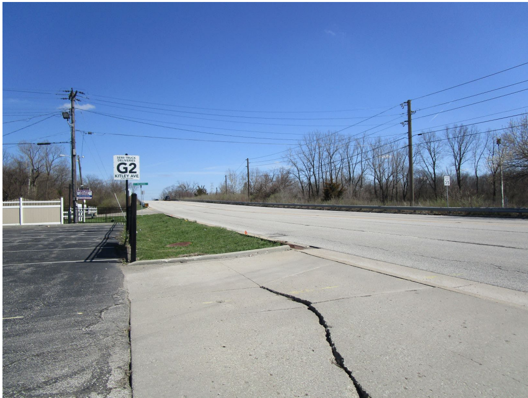
View looking east along Brookville Road
