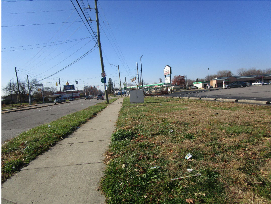
View looking east along Hanna Avenue
