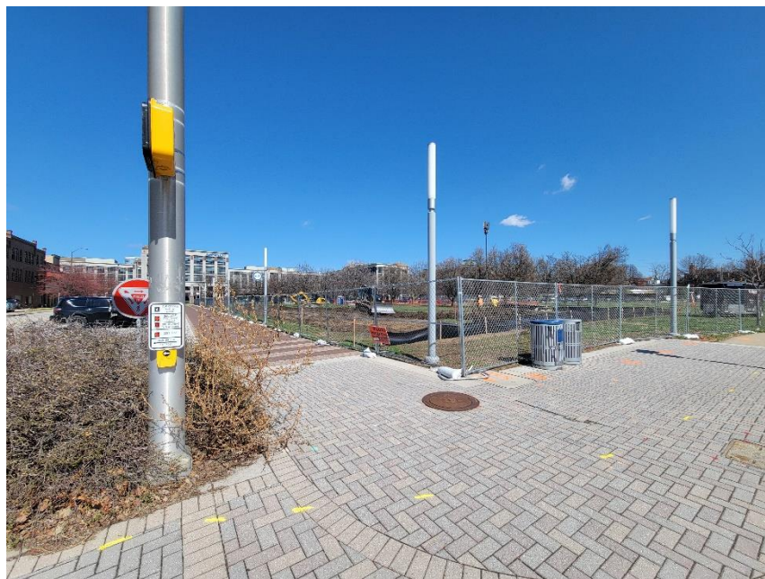
Photo 6: Subject Site Viewed from Southwest
