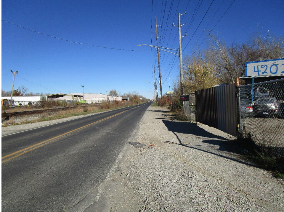
View looking northeast along railroad right-of-way and Massachusetts Avenue
