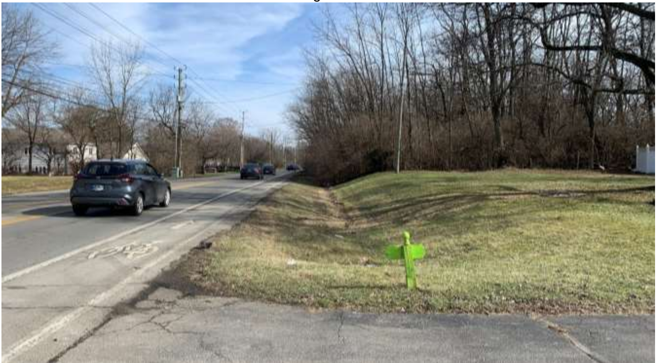
Photo of the street frontage east of the entrance drive.
