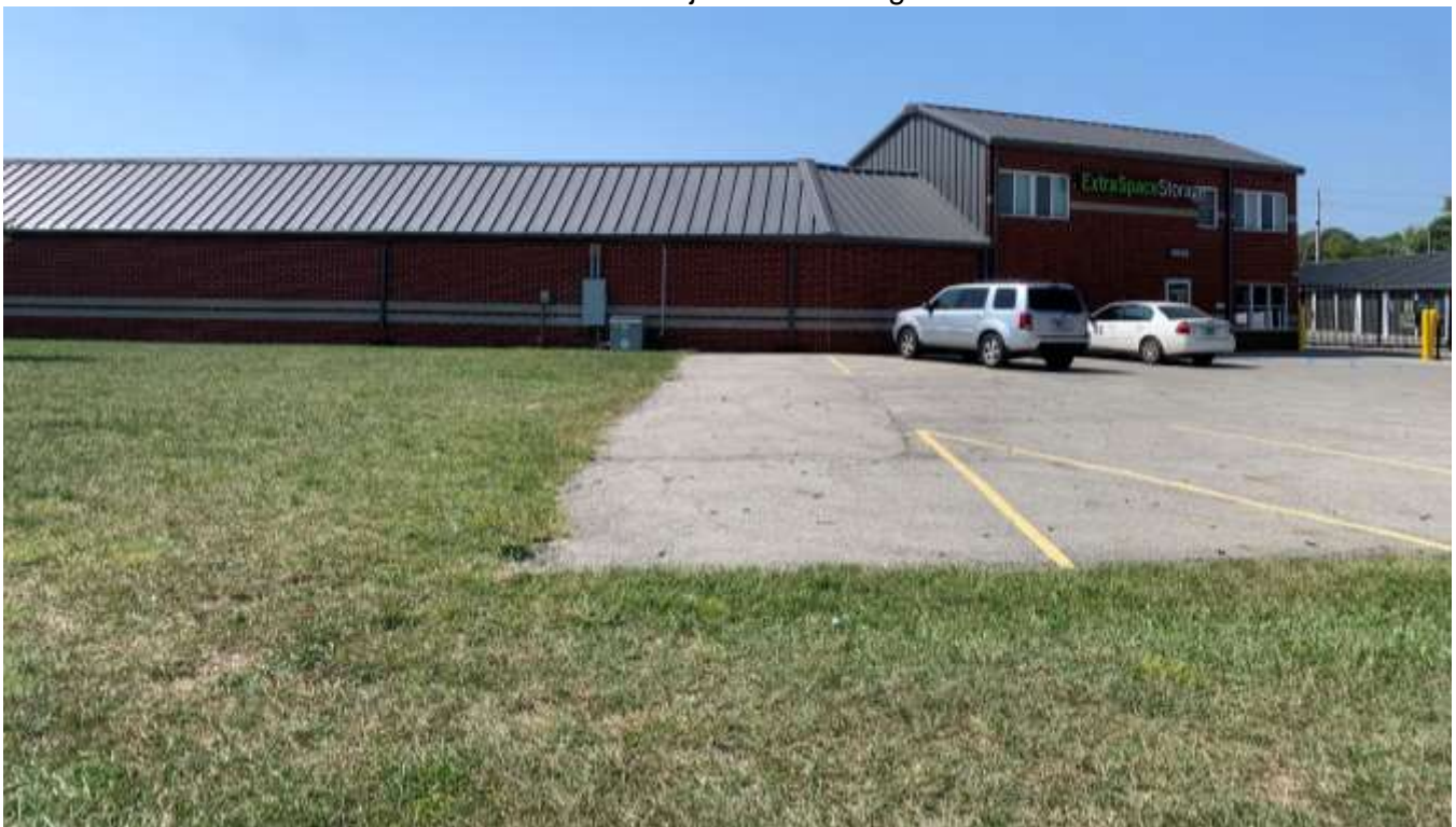
Photo of the subject site looking northwest.
