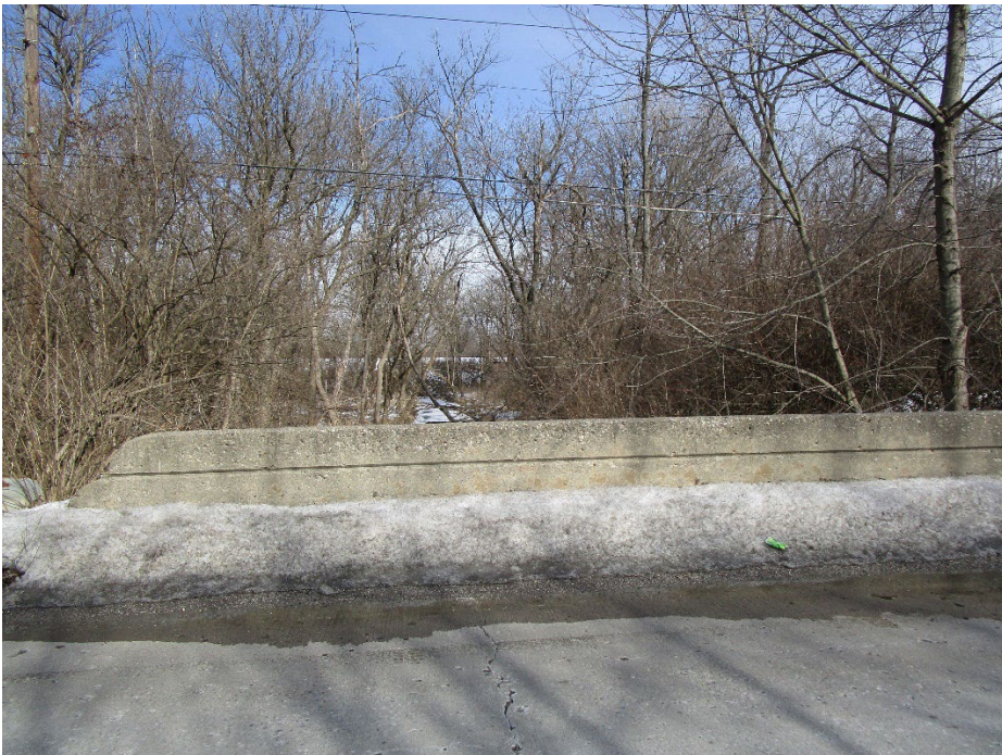
View looking east across South Shortridge Road along Fisher Branch
