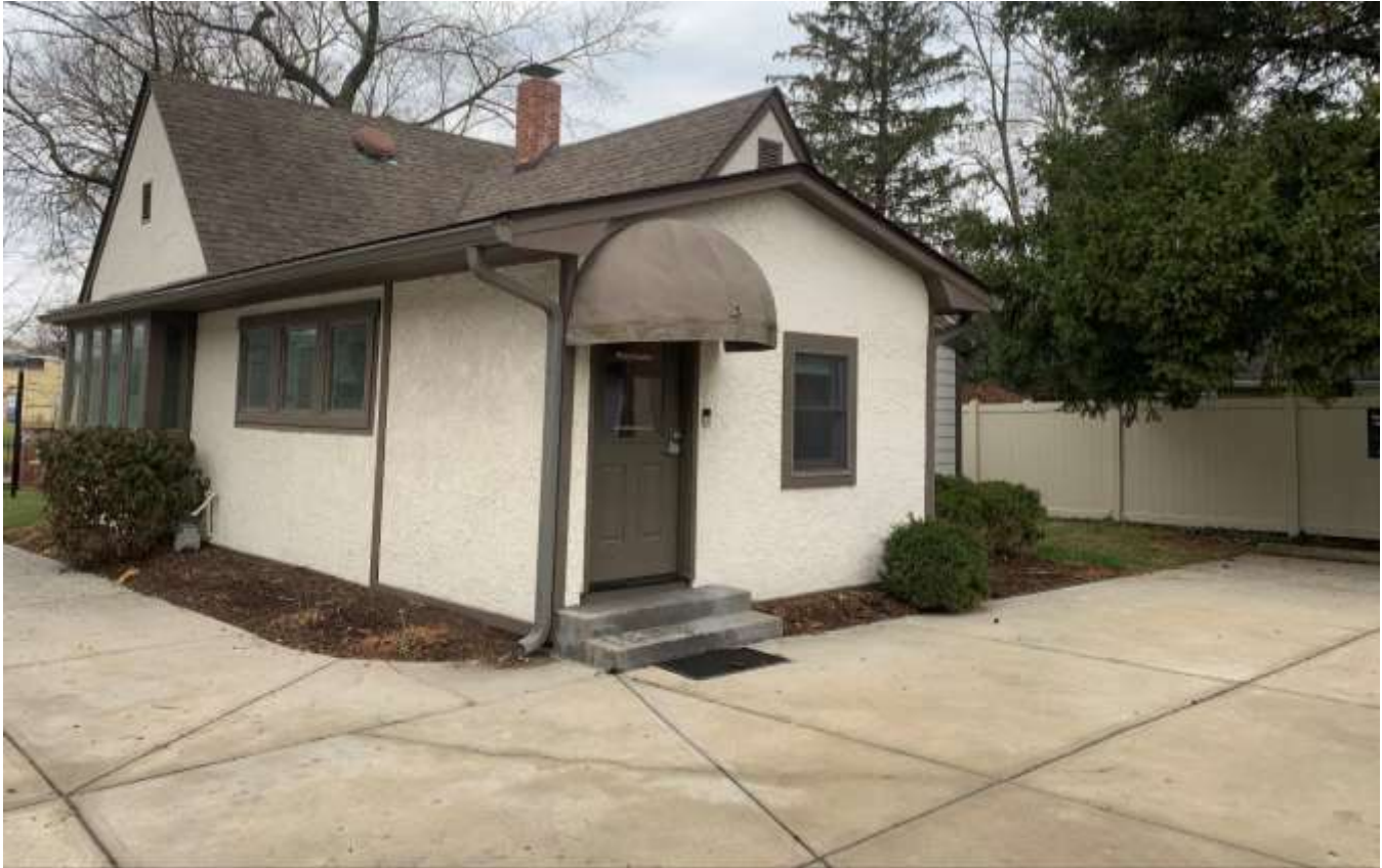
Photo of the rear entrance to the main building.
