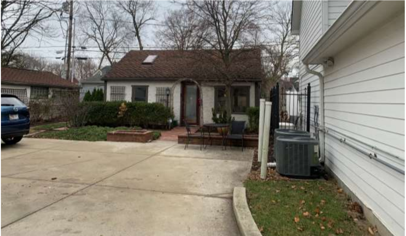
Photo of an accessory building on site.
