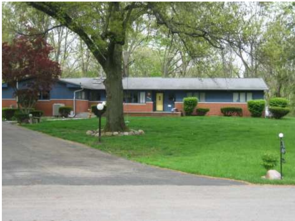
Photo fo adjacent neighbor to the west with complaint fencing, looking south.
