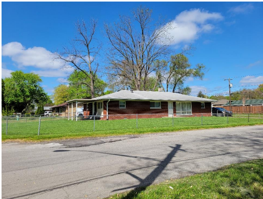
Photo 6: Adjacent Property to the Northeast
