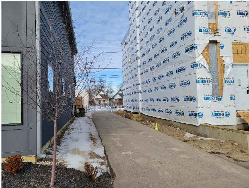
Photo 2: Existing Side Alley Viewed from South
