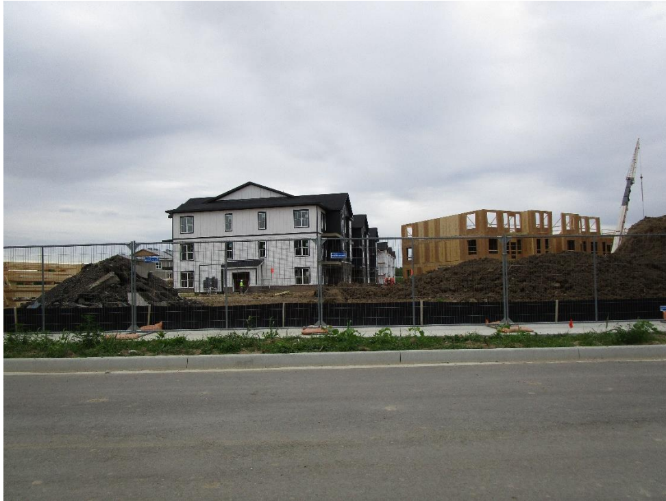
View of site looking east across Real Street
