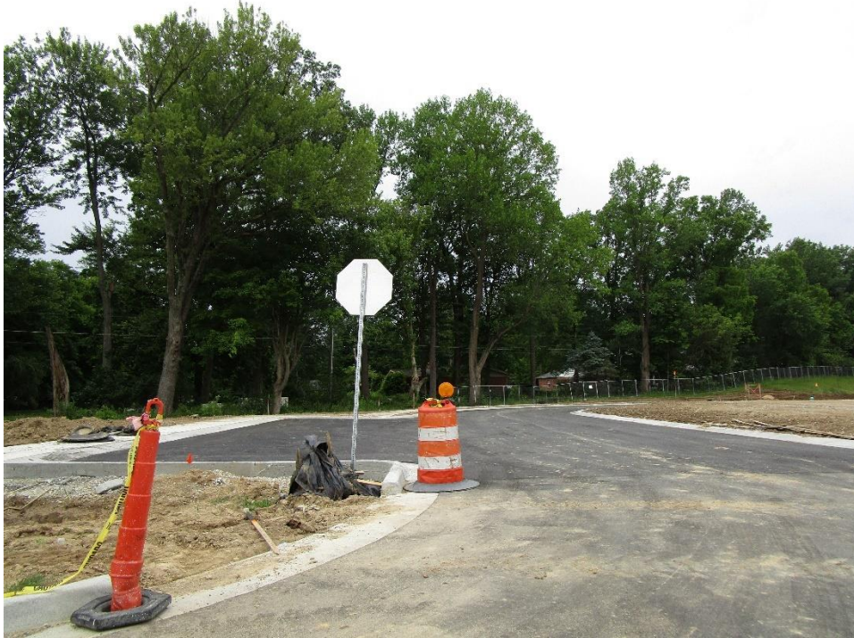
View from site looking southwest across Real Street
