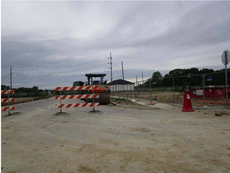
View looking north along Real Street
