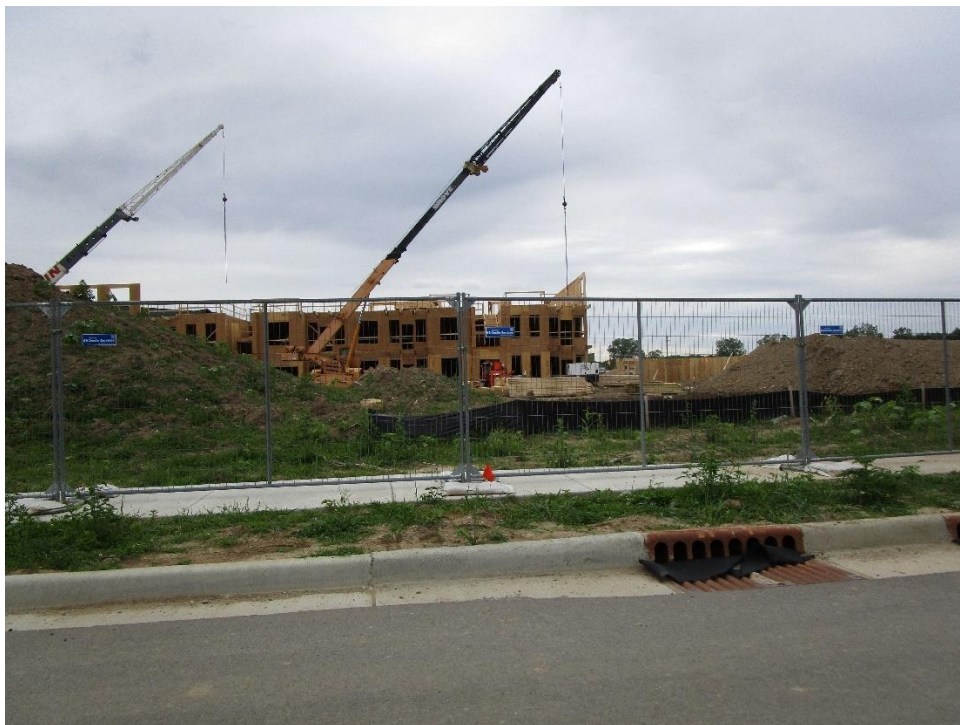
View of site looking north across Real Street
