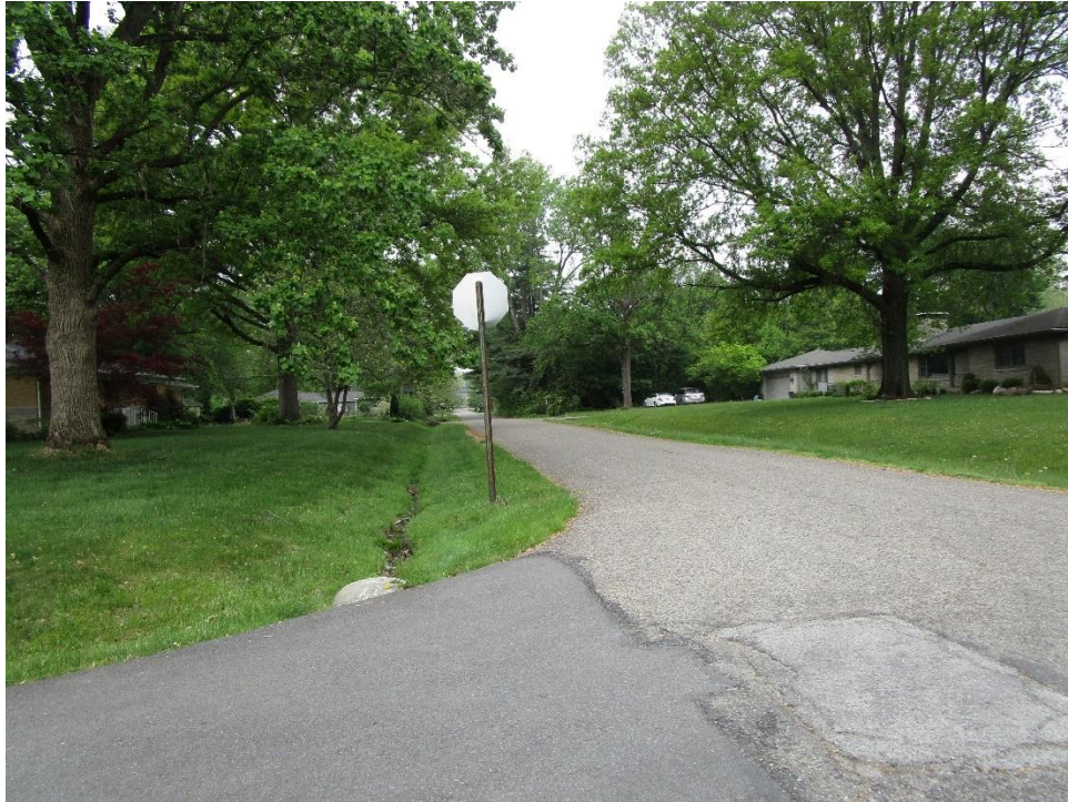
View looking north along Guildford Avenue
