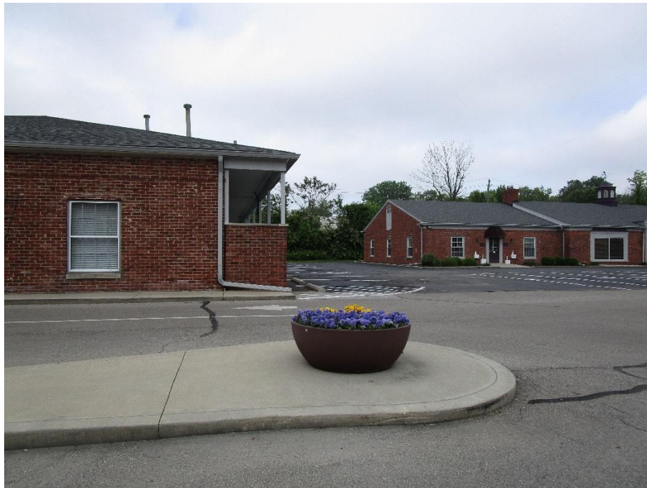
View of site looking west across entrance drive
