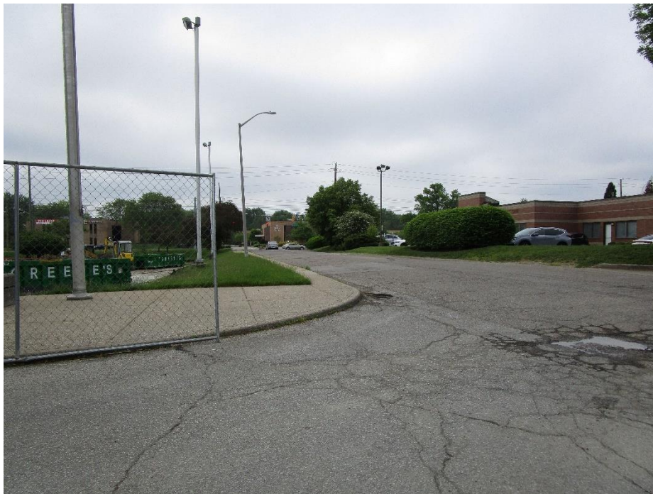
View looking south along Guildford Avenue
