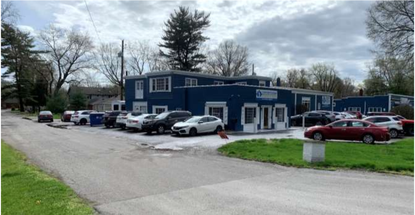
Photo of 7425 Westfield Boulevard looking southeast on the site.
