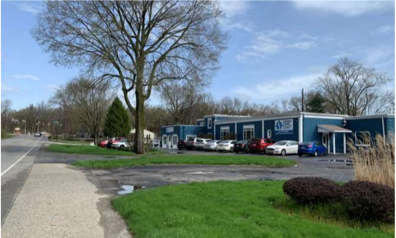
Photo of 7425 Westfield Boulevard looking north on the site.
