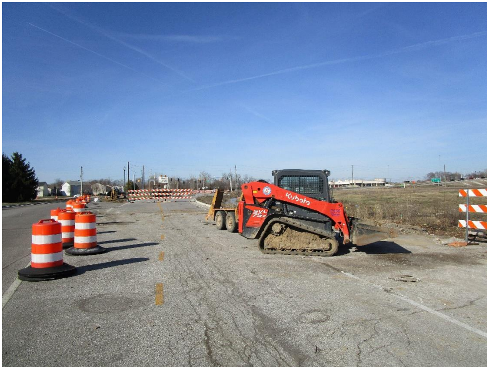
View looking north along Wellingshire Boulevard
