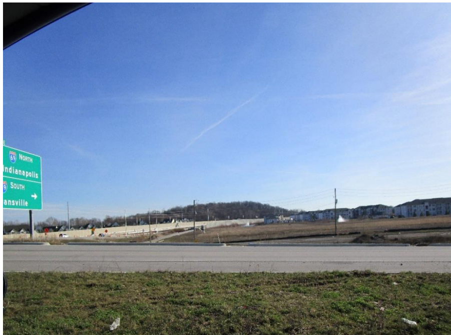
View of site looking south across West Southport Road
