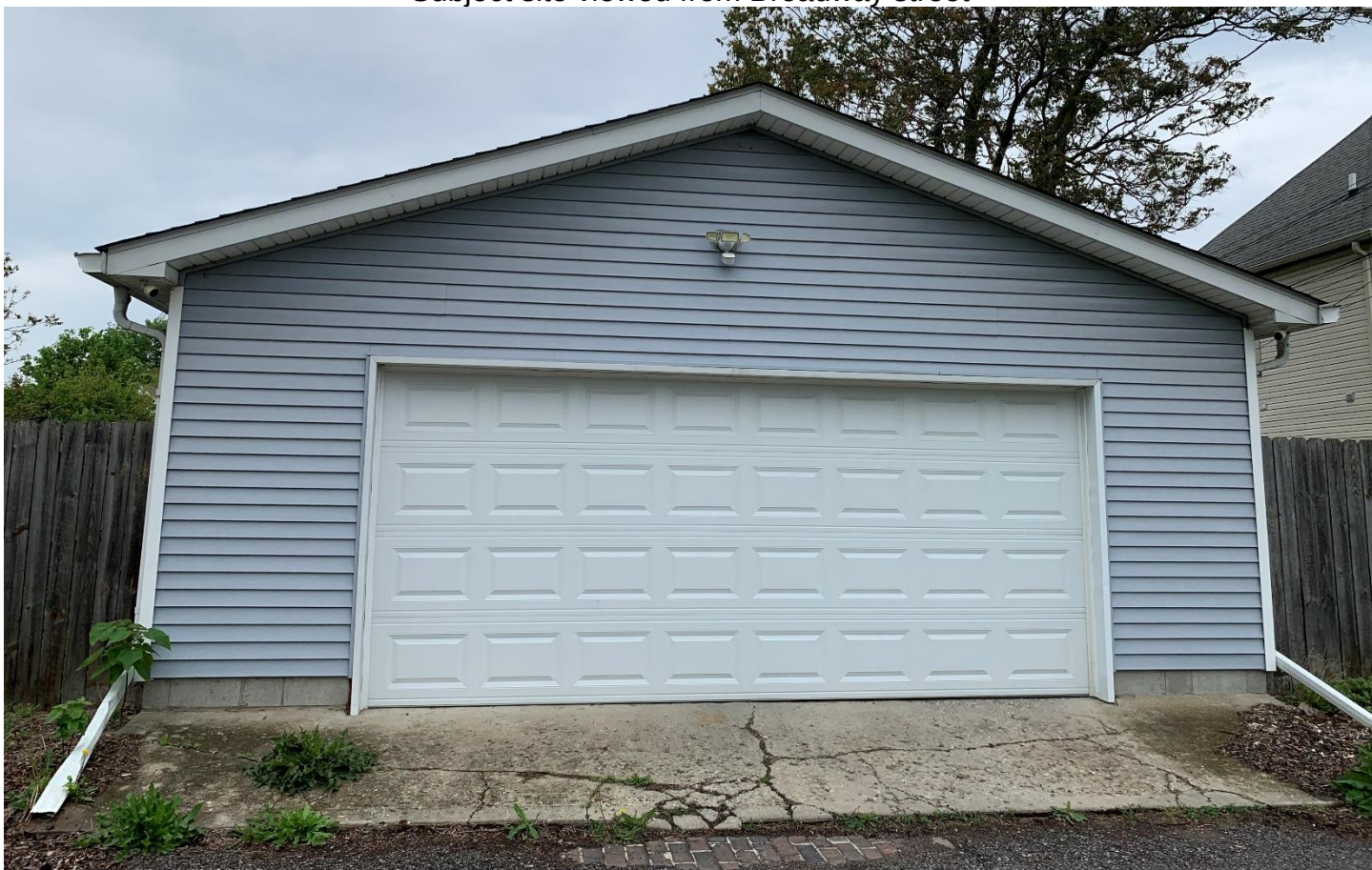
Existing garage 23.75 feet wide, to be demolished
