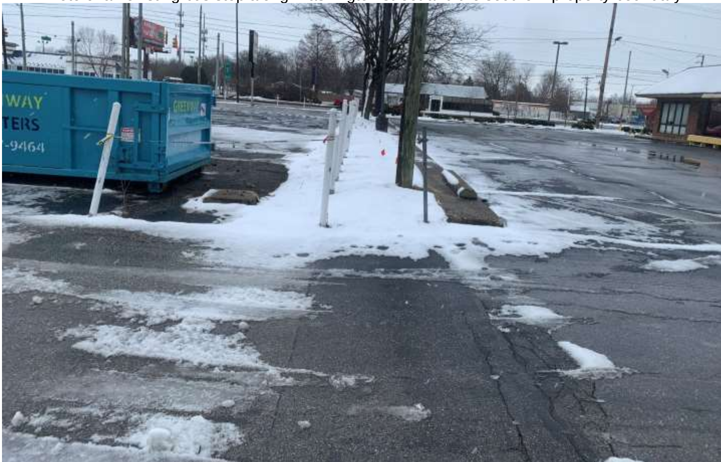
Photo of western property boundary looking south.
