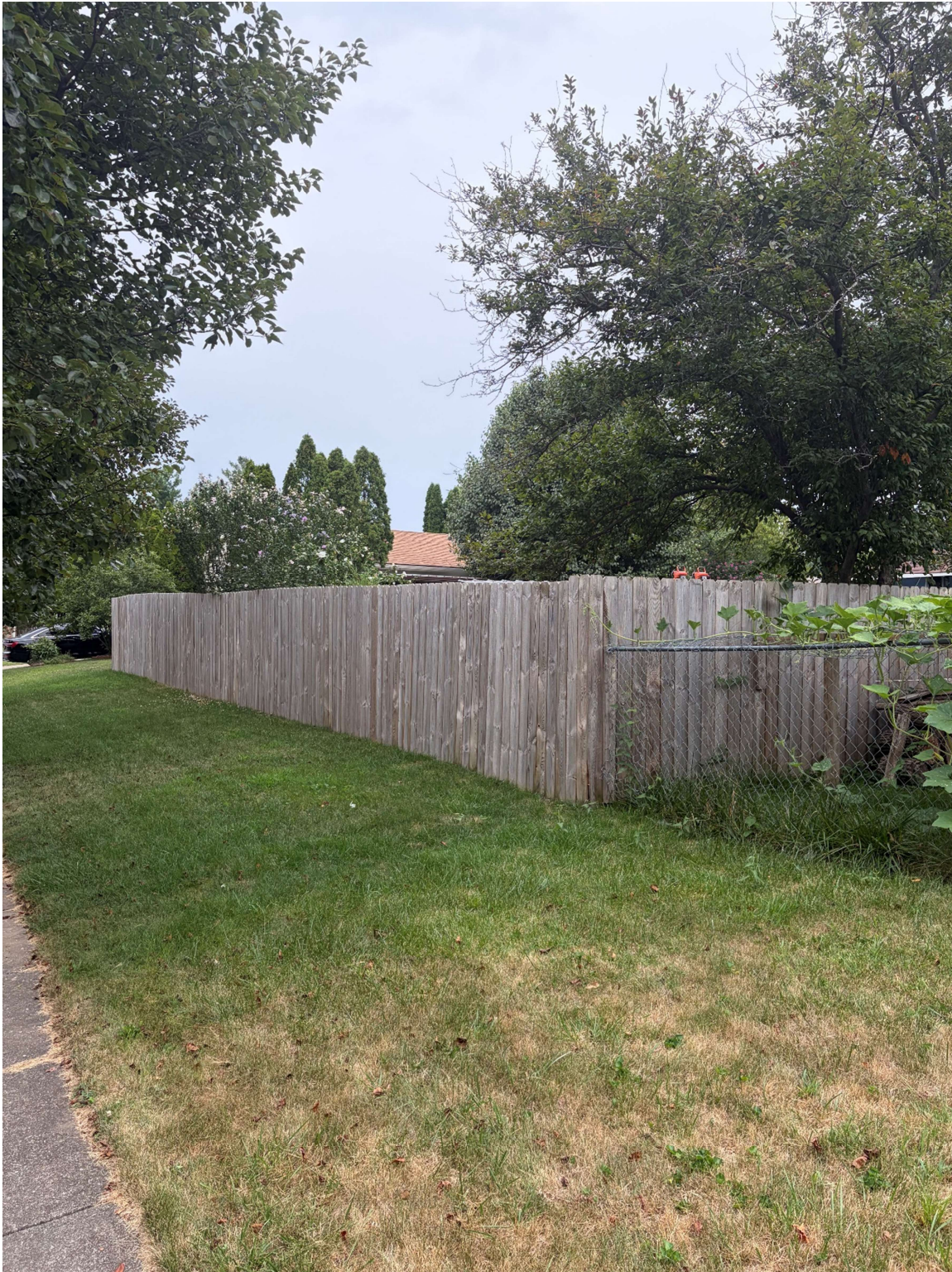
Figure 8 - looking North at fence
