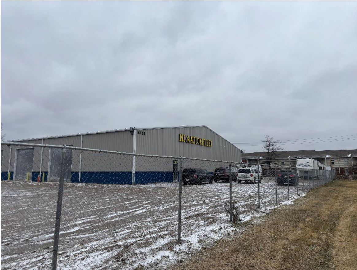
Figure 5 View of Sign
