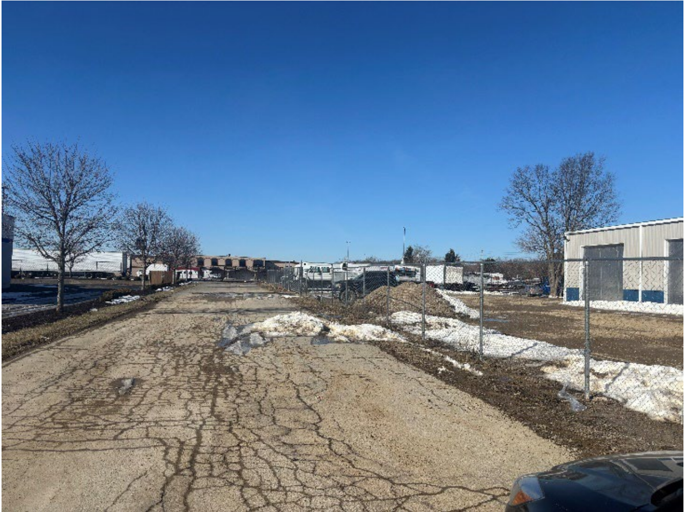
Figure 3 View west looking along the access road
