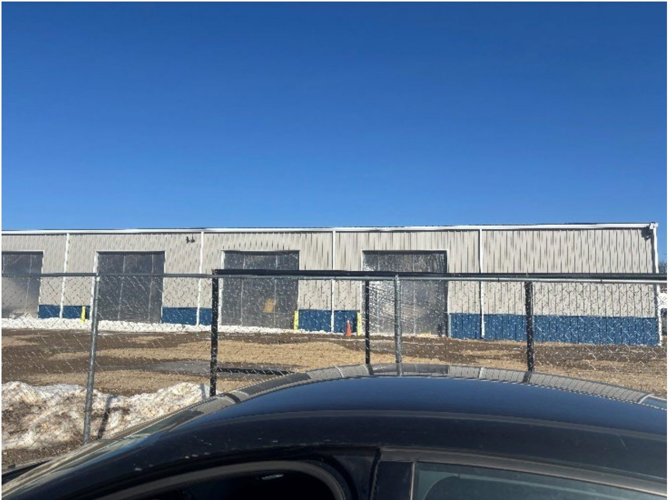
Figure 2 View of the subject building
