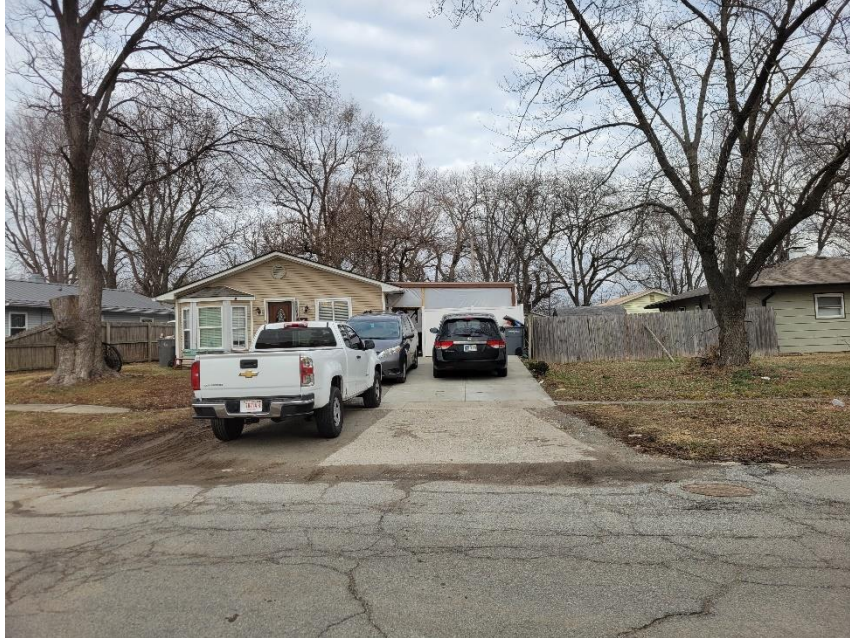
Photo 1: Subject Site Viewed from Southwest
