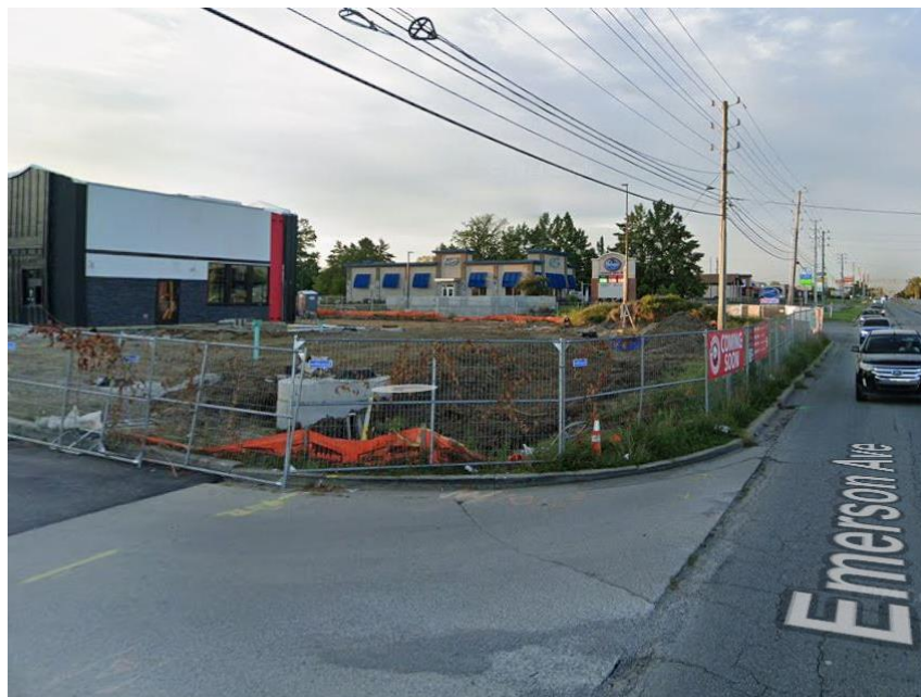
Photo 2: Subject Site from Northwest (September 2024)
