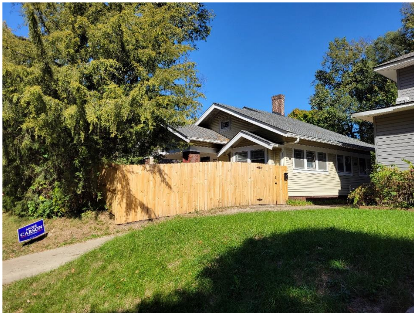
Photo 4: Subject Site Viewed from Southwest
