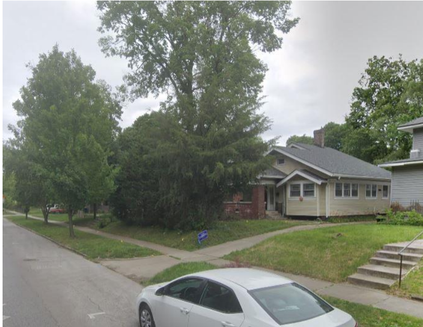
Photo 3: Subject Site Viewed from Southwest (June 2024)
