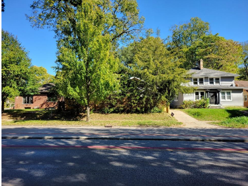
Photo 1: Subject Site Viewed from West (further sidewalk)
