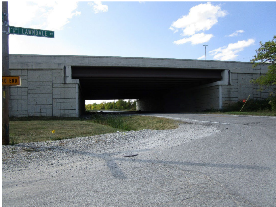
View looking northwest across intersection of Lawndale Avenue and West Minnesota Street
