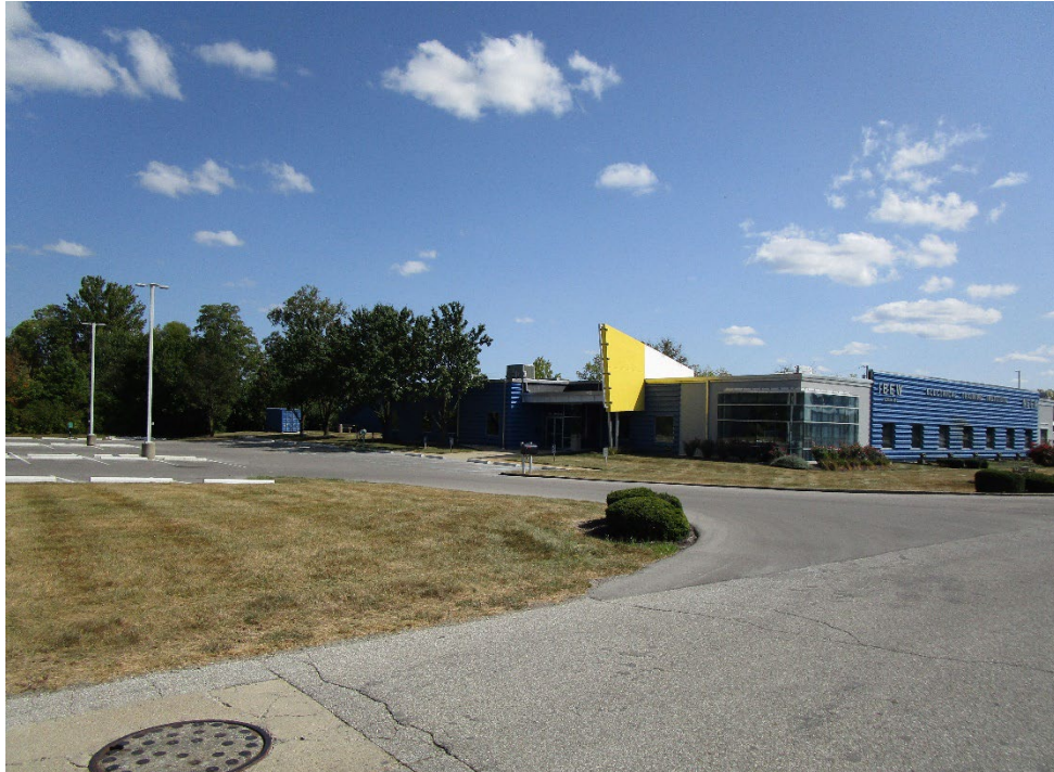
View of site looking southeast across Lawndale Avenue
