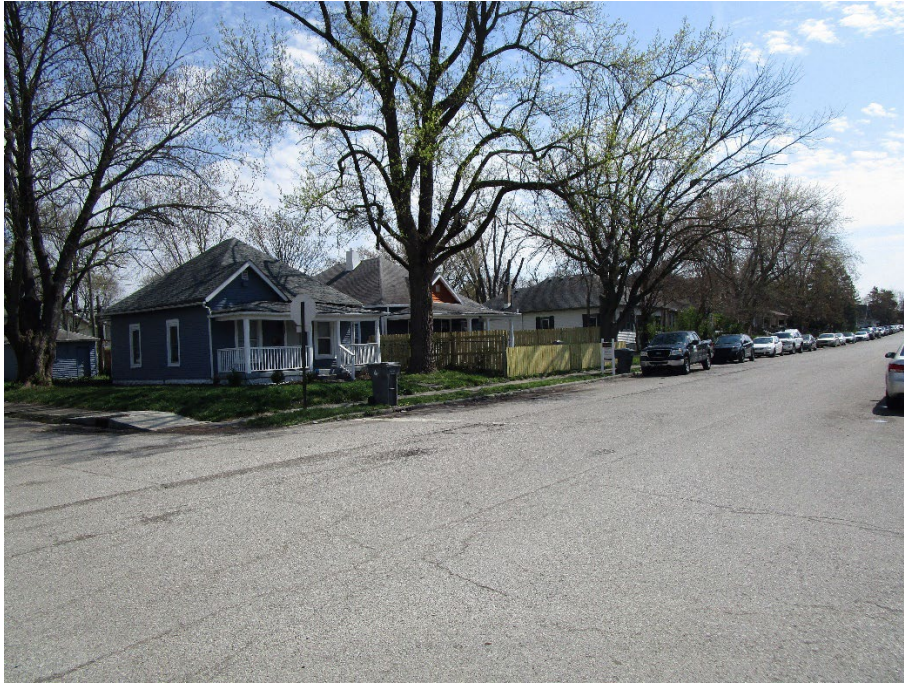
View looking southeast across intersection on North Olney Street and Nowland Avenue
