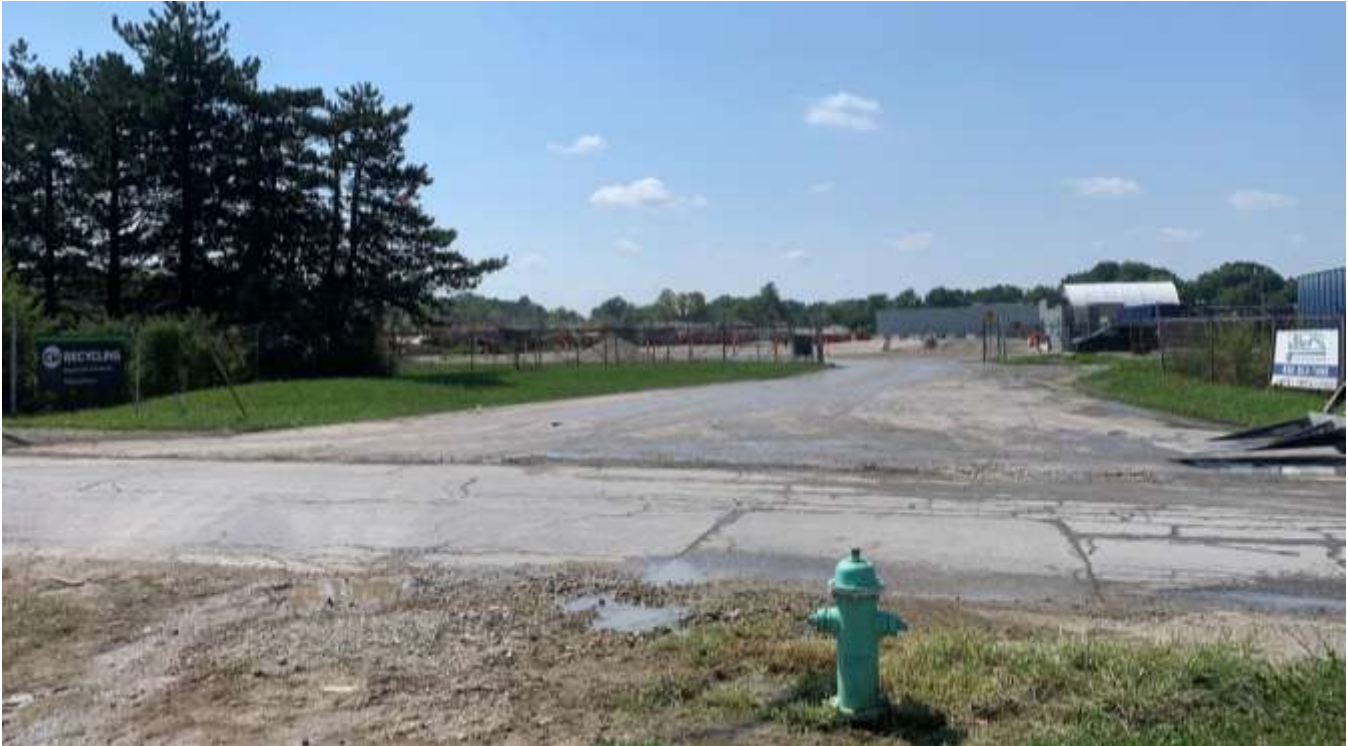
Photo of the existing driveway along 21 st Street.
