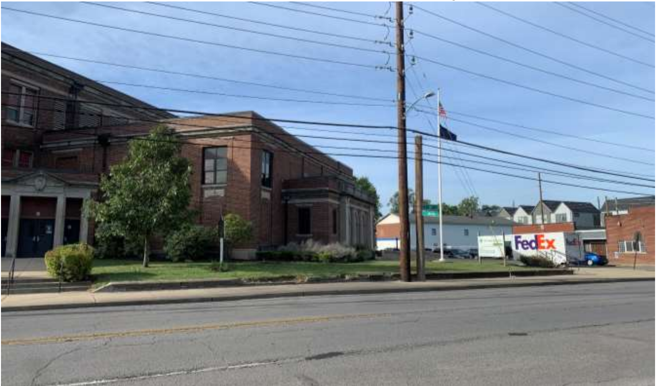
Photo of the school at 1301 East 16th Street looking southwest.
