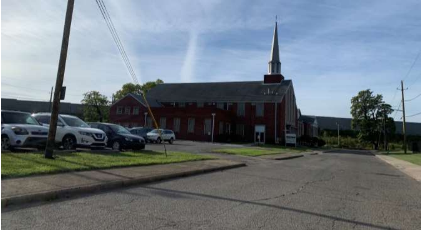
Photo of the church and associated parking east of the site.
