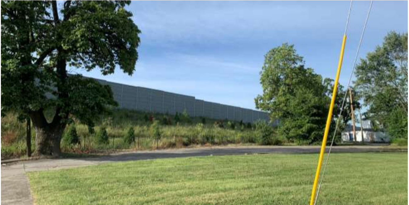
Photo of the southern property boundary at 1524 Dr A J Brown Avenue.
