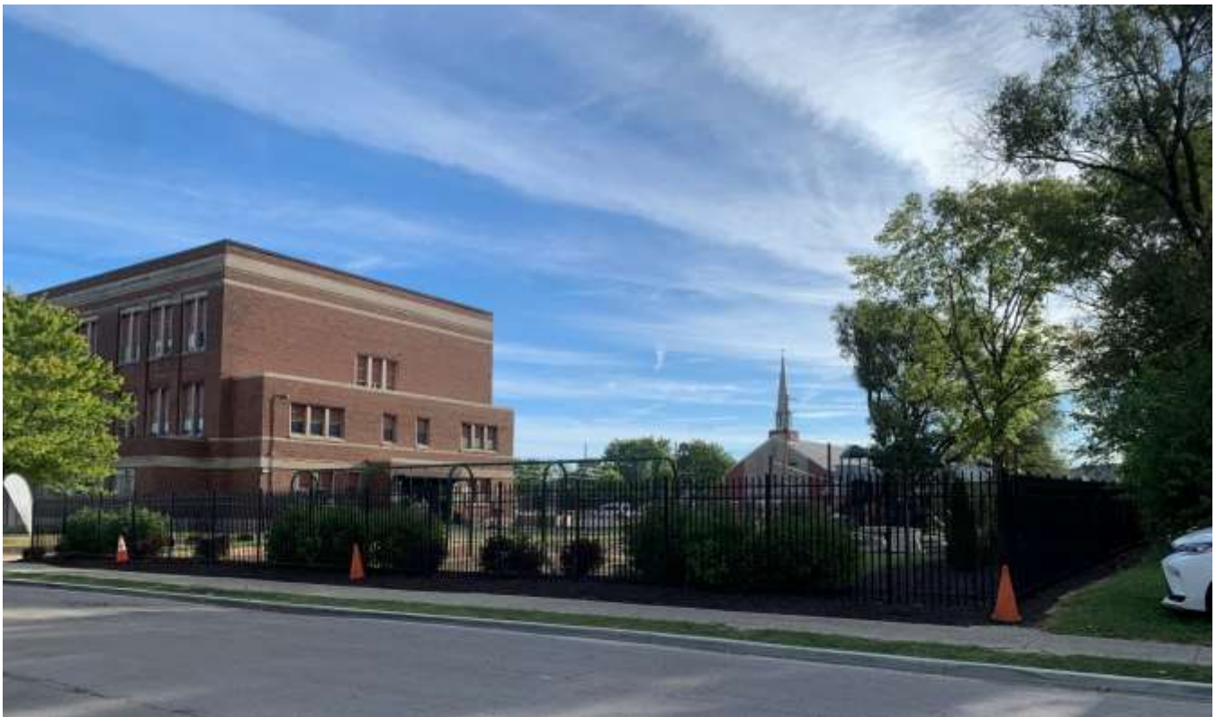
Photo of 1503 and 1517 Columbia Avenue developed with a playground.
