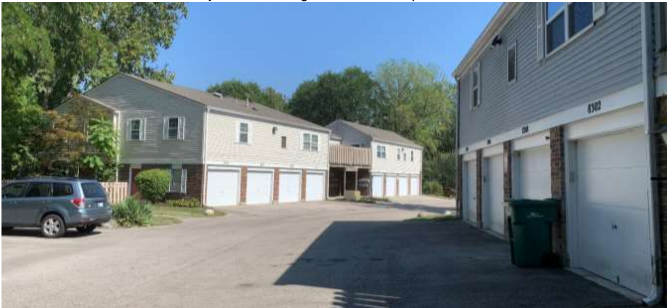
Photo of the quadrominiums southeast of the site looking southeast towards Woodall Drive.
