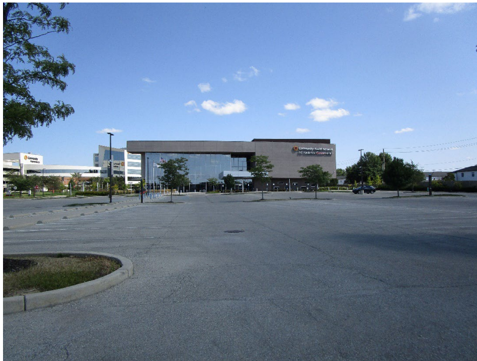
View of site looking north
